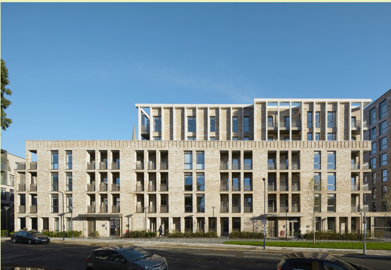
Unity Place by Gort Scott features a well-defined base, middle and top to create an attractive elevation with aligned and regularly spaced fenestration.
