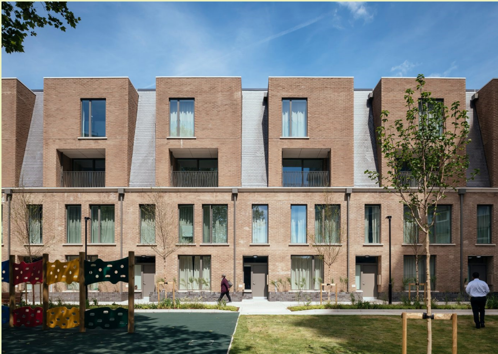
Agar Grove, Camden by Hawkins Brown is an example of a high quality residential development in an urban location which is Passivhaus accredited.
