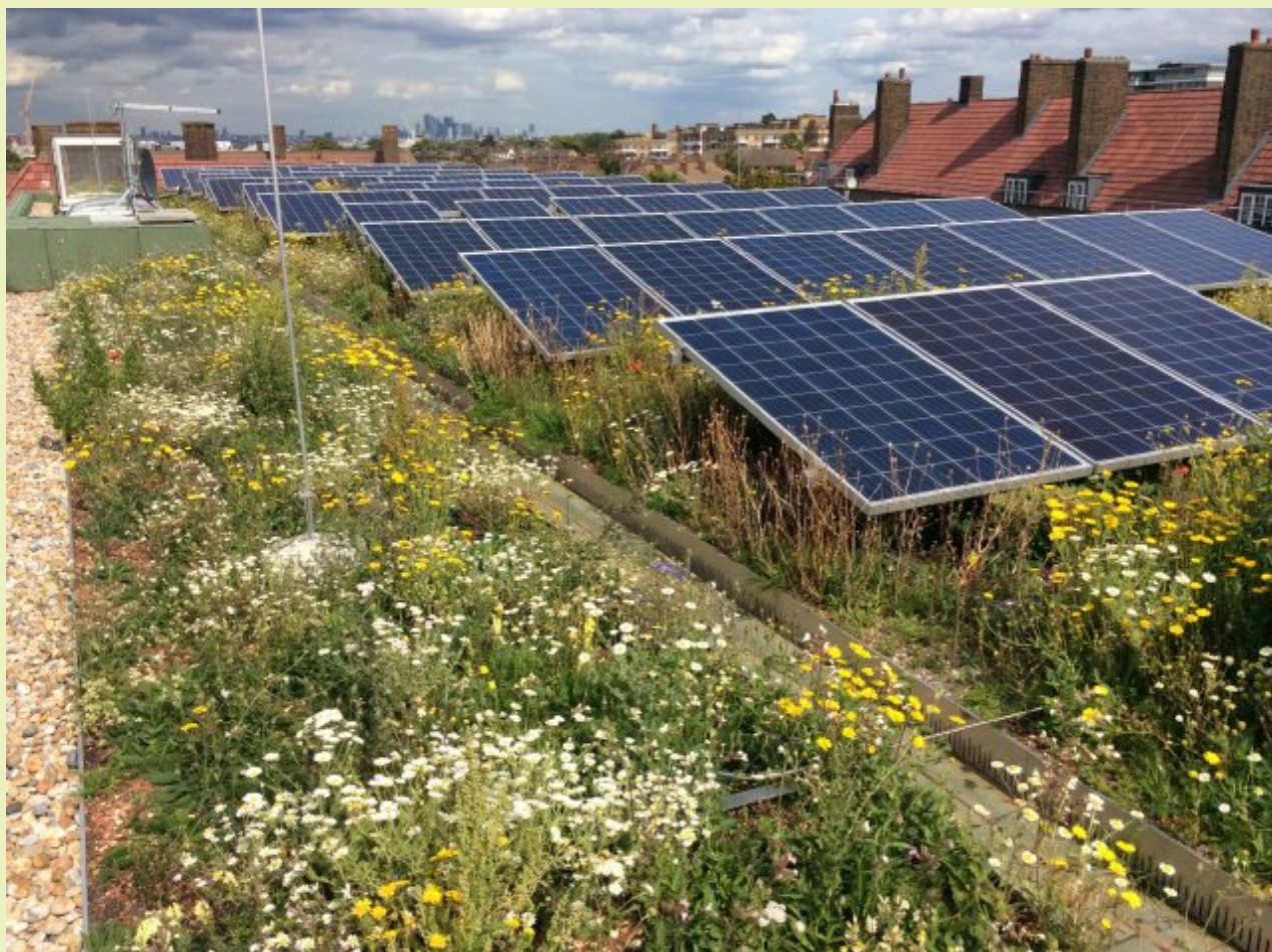
An example of a biosolar roof. Greening and solar panel provision for heating and hot water can be co-located on roofspace.
