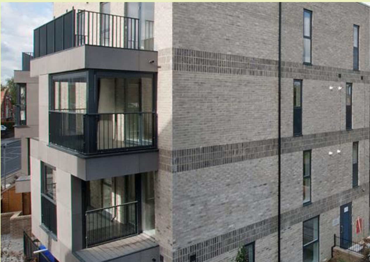
Architectural features can positively enhance buildings and the areas they sit within. This flank elevation to Greenstock Lane features stack-bonded brick banding, enlivening what would otherwise be an overly plain elevation.
