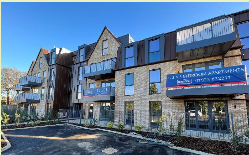
This residential development in Hatch End features contextually sympathetic roof forms and three-storey shoulder massing stepping up to four storeys for central portions.
