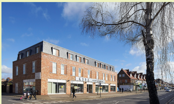
Sycamore Court, Harrow is an example of a low-density mixed use development with a Cash and Carry on the ground floor and housing above.
