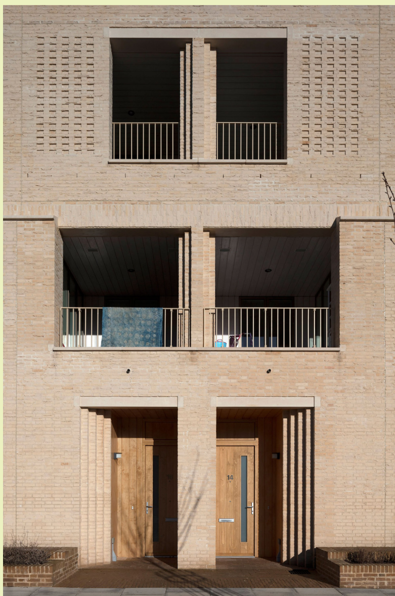
Kings Crescent Estate by Karakusevic Carson Architects features a wealth of architectural detailing to create visual interest and add depth to elevations, with stepped brickwork creating deep and sheltered reveals for front doors and private balconies aligning with other elements of the elevation.
